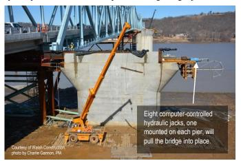
on the slide plates to grease the skids. Then, through a series of grabs and pulls, the bridge will be slid into place. Each grab and pull is expected to move the bridge 20–22 inches – up to 10 feet per hour.
